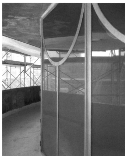
Fig. 3. Exterior view of existing original third-floor steel-frame glass walls, photograph 2006.
