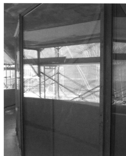
Fig. 4. Exterior view of storm window with insulated-glass units installed during a c. 1994 in-house retrofit, photograph 2006. The exterior glazing obscured the original steel frame.
