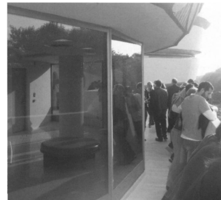
Fig. 8. Exterior view of new thermally broken steel-frame glass walls installed on the fourth floor, photograph 2009.
